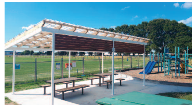
The completed shelter.
