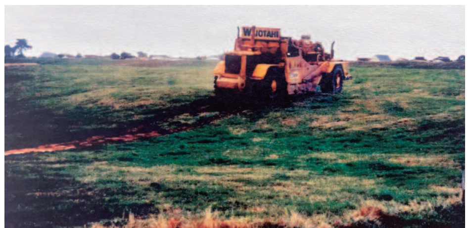
The first tractor gets work underway.
